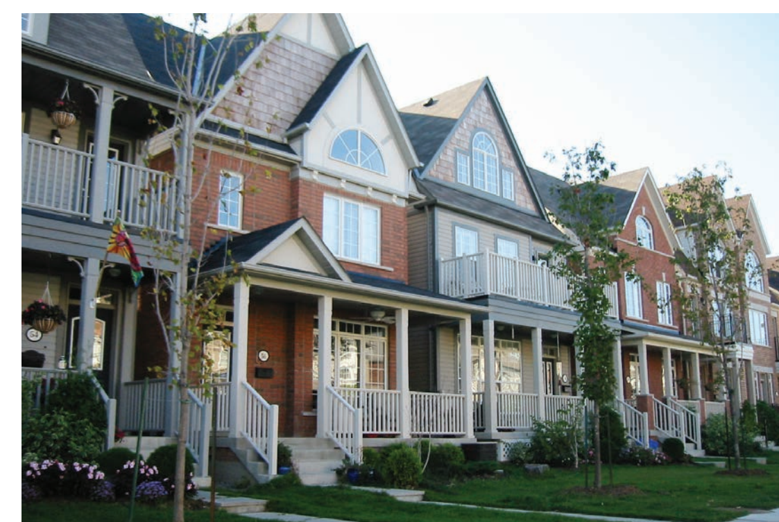
Low to mid-rise residential buildings
