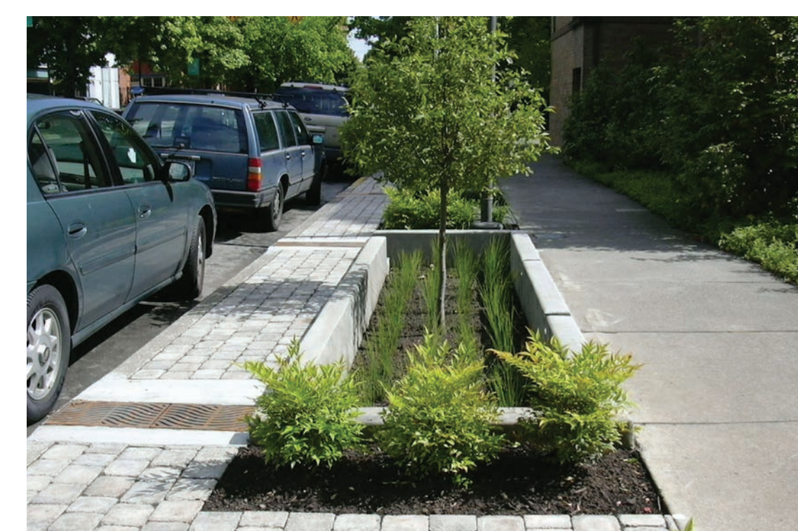
Boulevards designed for stormwater retention
