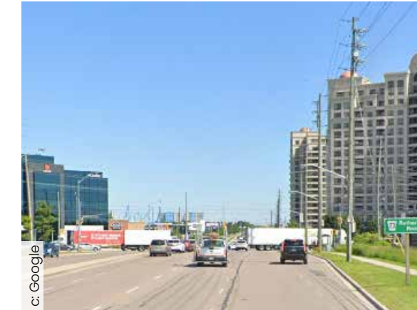
Fig. 24. Aboveground utilities along Jane Street.
