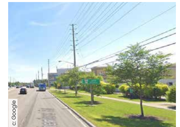
Fig. 25. Aboveground utilities along Rutherford Road.
