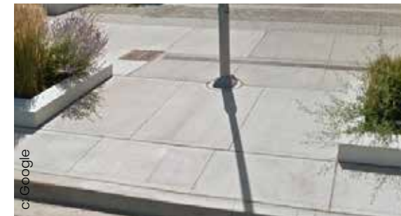
Fig. 123. Poured in place concrete with sawcut jointing.
