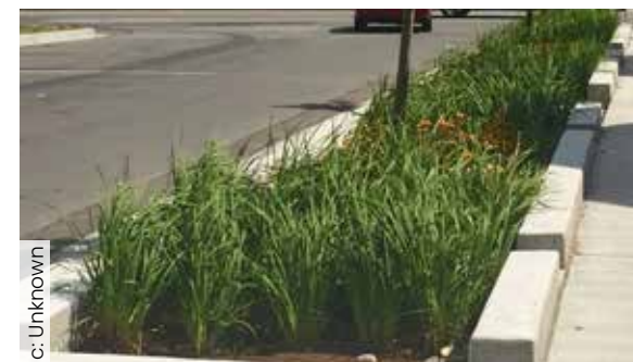
Fig. 96. Bio-retention / storm planters.
