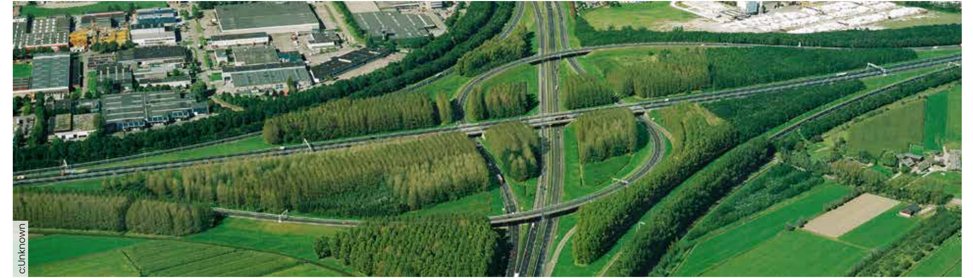
Fig. 76. Greening of the Highway 400 right-of-way.
