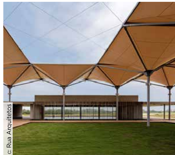
Fig. 88. Example rainwater harvesting canopy.
