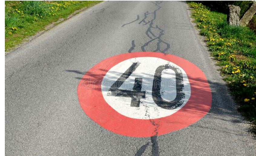
40 Km/H Pavement Marking
