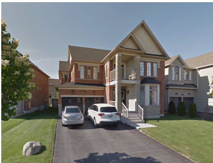
On lots with a minimum width of 15 metres, the garage should be recessed from the front wall of the house, and the width of the garage should not be greater than the width of the house. (Guideline 4.17)
